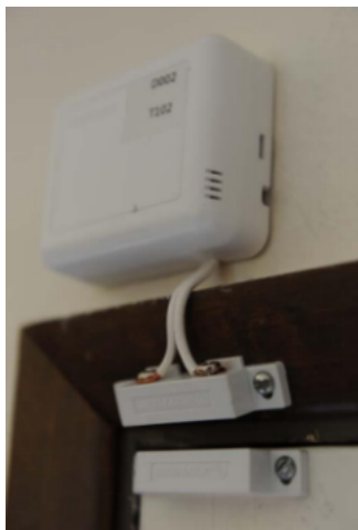
Figure 6.4: A CASAS door sensor, which detects whether a door is open or closed.
