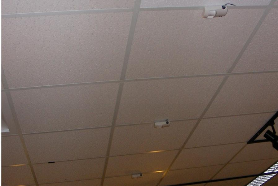
Figure 2: Sample of PIR motion detectors, as installed in the Tokyo testbed.
