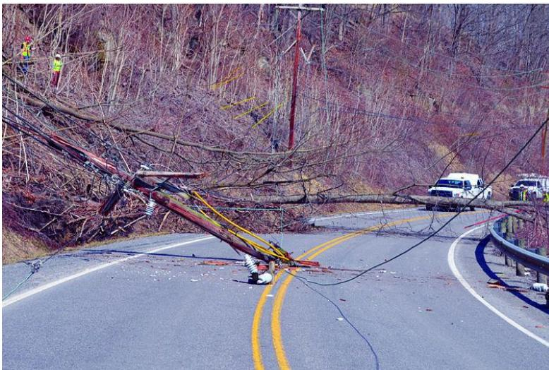
Fig. 2.4.9. Landslide damage to a power line. The Exponent Telegram <http://www.theet.com>. Staff photo by Darlene J. Swiger
