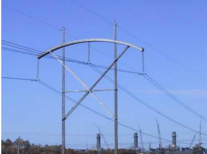
Fig. 2.2.8. Overhead shield wires visible at the tops of the two poles. (courtesy J.R. Stewart)
