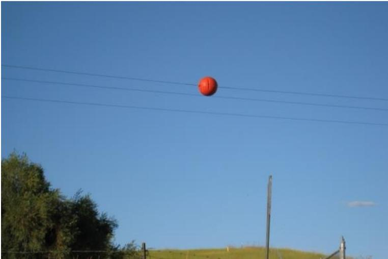
Fig. 2.2.23. Marker ball on power line conductor near an airport.
