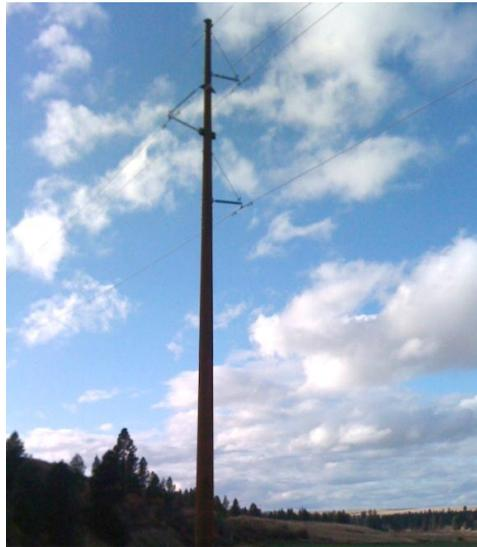
Fig. 2.2.12. Transmission line tower with line post insulators. These do not allow movement of the conductors in any direction. Hence, clearances between conductors and the tower can be smaller.
