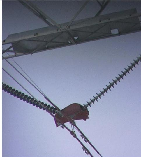
Fig. 2.2.24. Bird control hardware. (courtesy A. Stewart, EDM Intl.)
