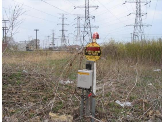
Fig. 2.3.2. Although not evident because most pipelines are buried, there is a buried pipeline to the left of the transmission line in this photo. (courtesy, J. Dabkowski)
