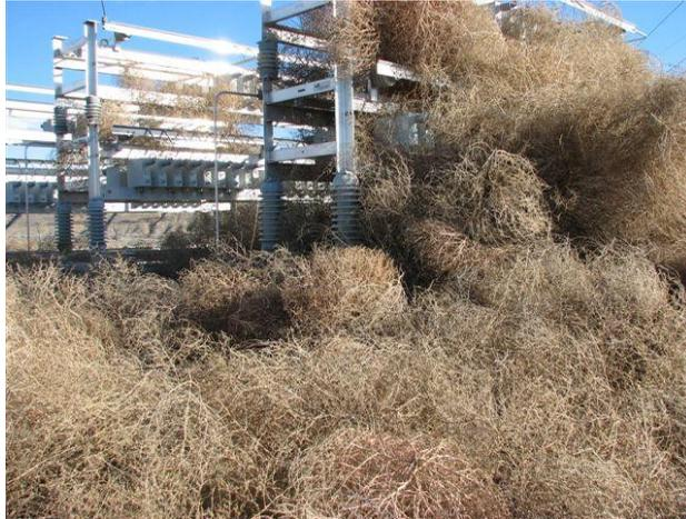
Fig. 2.4.12. Windblown tumbleweeds in a substation. (Courtesy of BPA)
