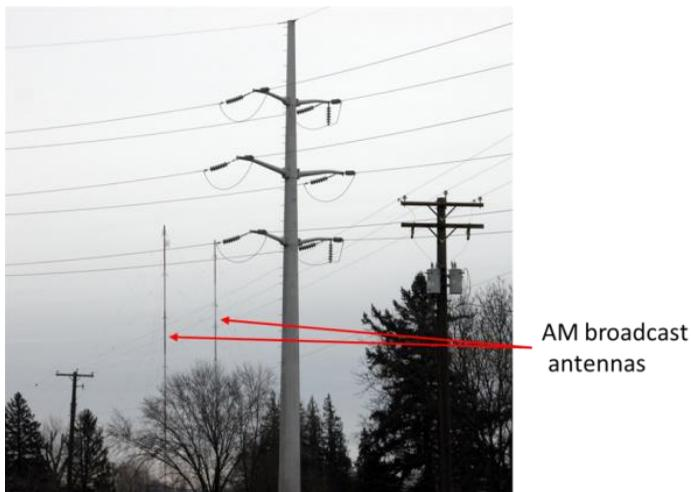
Fig. 2.3.7. Transmission line with nearby AM transmitting antennas in background. (courtesy T. Osborn, BPA)
