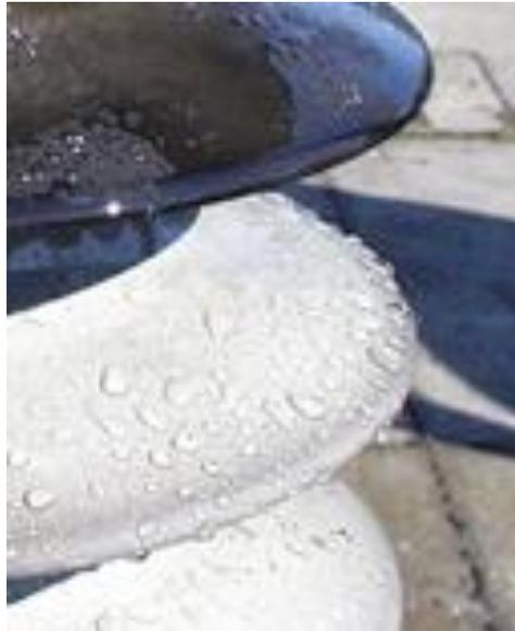
Fig. 2.4.3. Rain on a transmission line insulator. (<http://www.bing.com/images/>)
