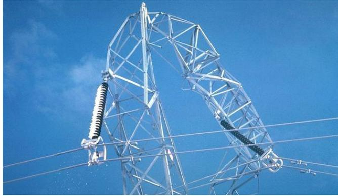
Fig. 2.4.1. Iced insulators after a snowstorm resulting in tower failure. (courtesy BPA)
