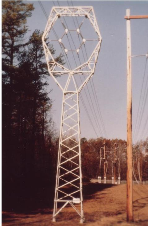
Fig. 1.7.2. Experimental six-phase power system tower. (Courtesy J. R. Stewart)
