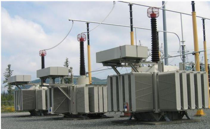
Fig. 2.2.30. A three phase shunt reactor installed in a substation. (courtesy BPA)
