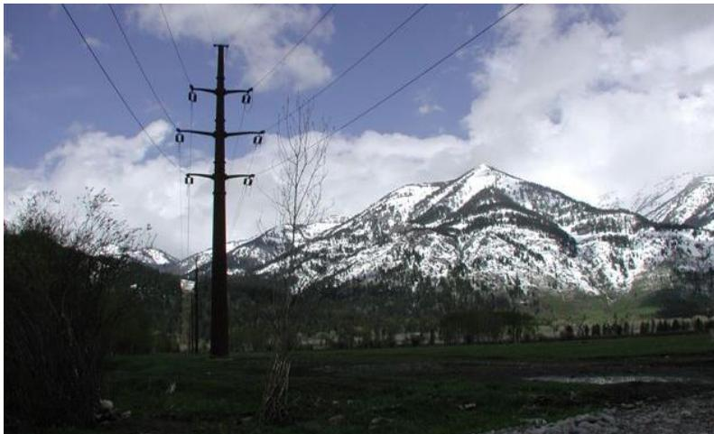
Fig. 2.2.9. Double circuit transmission line. (courtesy R. Aho, BPA)
