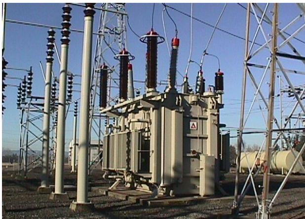
Fig. 2.2.32. Three phase 230 kV – 115 kV power transformer. (courtesy BPA)
