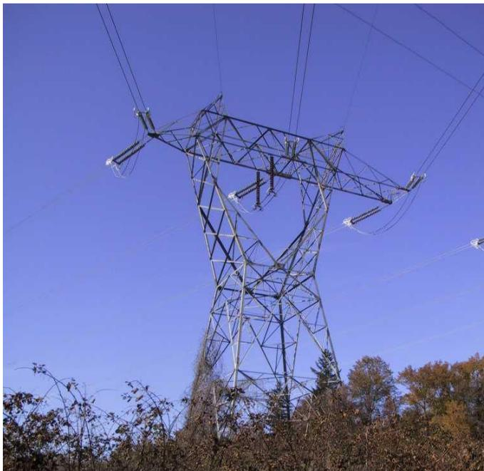
Fig. 2.2.15. A “heavy angle” structure at a change in the transmission line direction.
