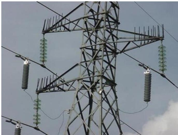
Fig. 2.2.28. Three line surge arresters installed along a transmission line, each connected from an individual phase to ground. <http://www.liveline.co.za/high-voltage-surge.php>
