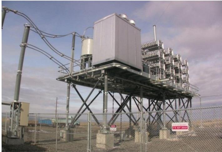
Fig 2.2.27. Series capacitors along a 500 kV transmission line. (courtesy J. Hildreth, BPA)
