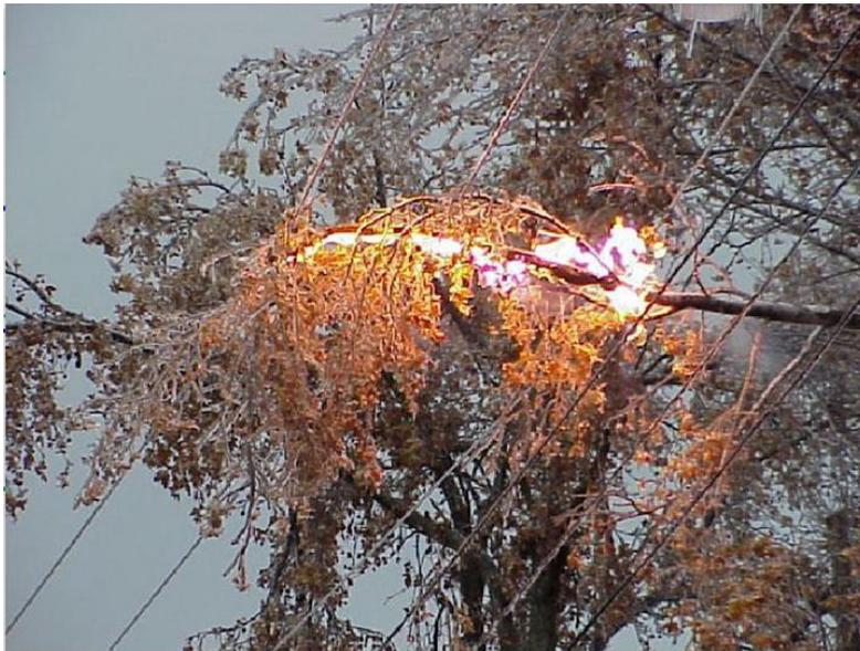
Fig. 2.2.18. Flashover to vegetation from a power line. Although this photo is from a lower voltage distribution line, it illustrates the point that vegetation can cause faults. (courtesy C. Gellings, EPRI)
