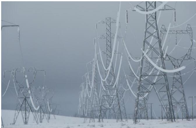
Fig. 2.4.2. Iced conductors in a winter storm that caused conductors to sag. (courtesy BPA)
