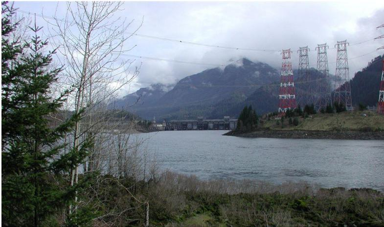
Fig. 2.2.19. River crossing that requires special towers for long spans. (courtesy R. Aho, BPA)
