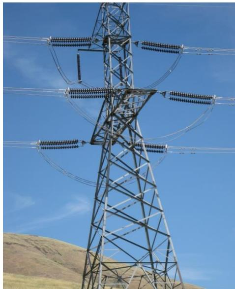
Fig. 2.2.11. A dead end tower that is stronger and does not allow conductor movement parallel to the transmission line direction
