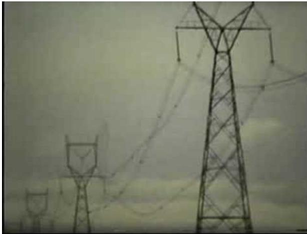
Fig. 2.4.6. Conductor galloping in wind <http://i.ytimg.com/vi/IfhfsjFG0jo/0.jpg>
