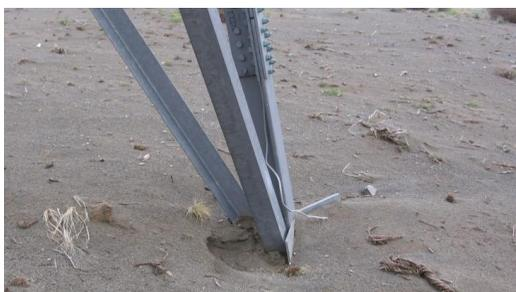
Fig. 2.2.25. Wire connection to tower ground. (courtesy N. Mullen, BPA)
