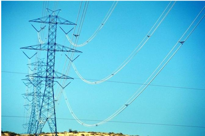
Fig. 2.2.14. A sagging conductor. (courtesy BPA)
