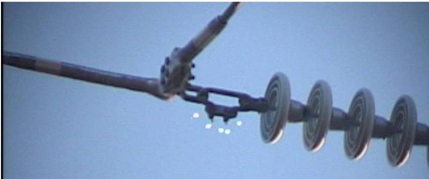
Fig. 1.6.2. The white spots at the tips of the attachment hardware are corona discharges. (courtesy B. Clairmont – EPRI)
