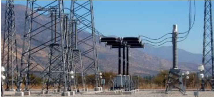
Fig. 2.2.31. A three phase circuit breaker installed in a substation.
