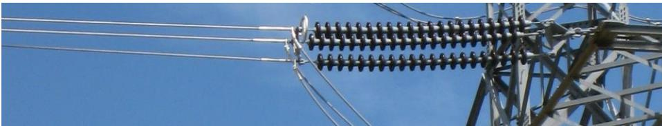
Fig. 2.2.6. A three conductor bundle on a 500 kV line
