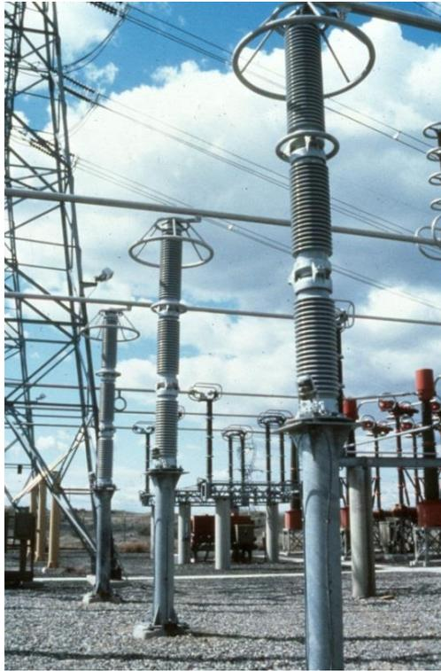
Fig. 2.2.29. Three single phase surge arresters installed in a substation. (courtesy of BPA)
