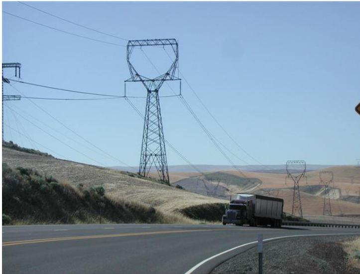
Fig. 1.7.1. Transmission line structure for the HVDC Pacific Intertie. (courtesy R. Aho, BPA)
